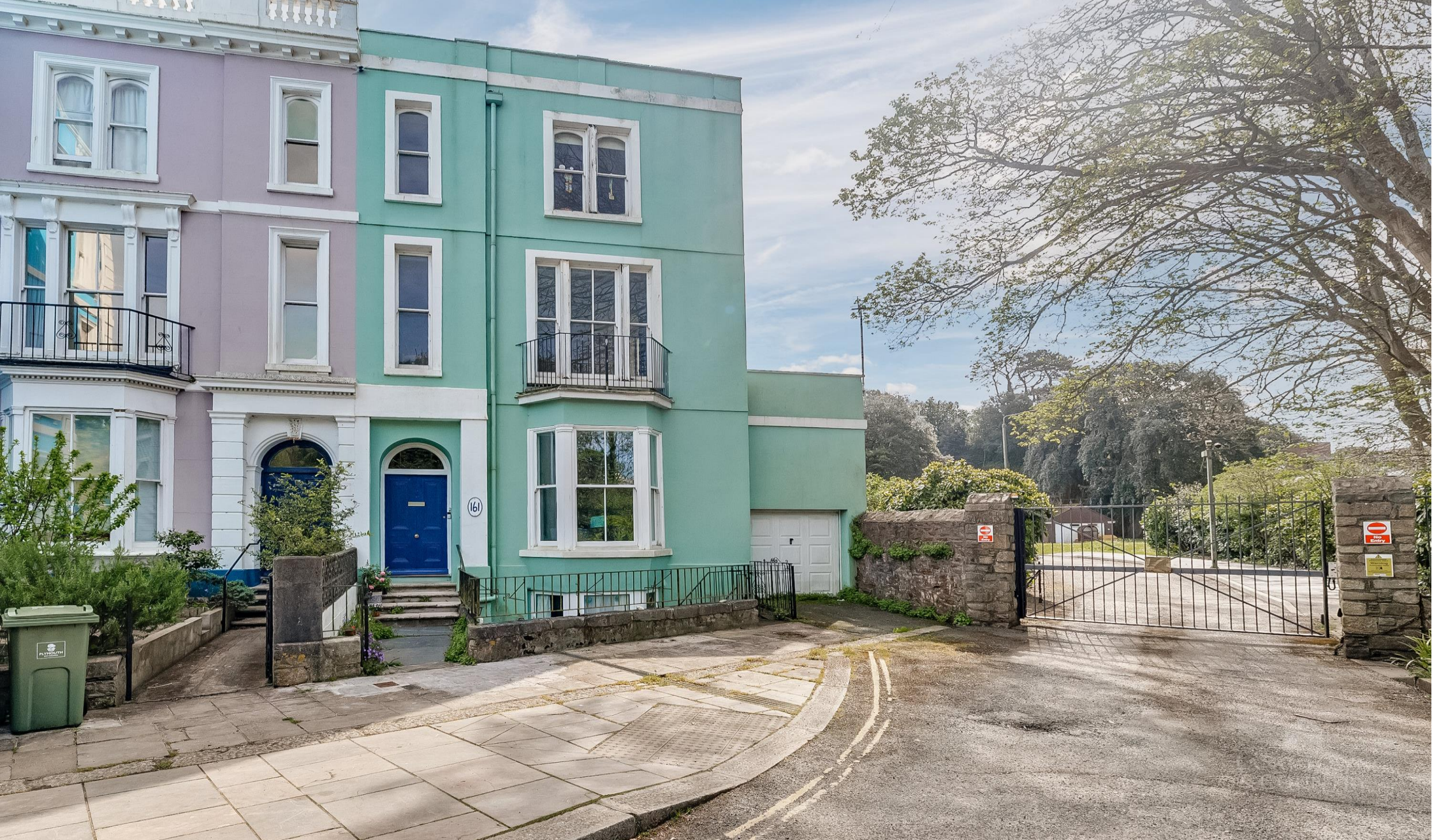
161, Ground & First Floor Maisonette, Durnford Street, Stonehouse, Plymouth, PL1 3QR
