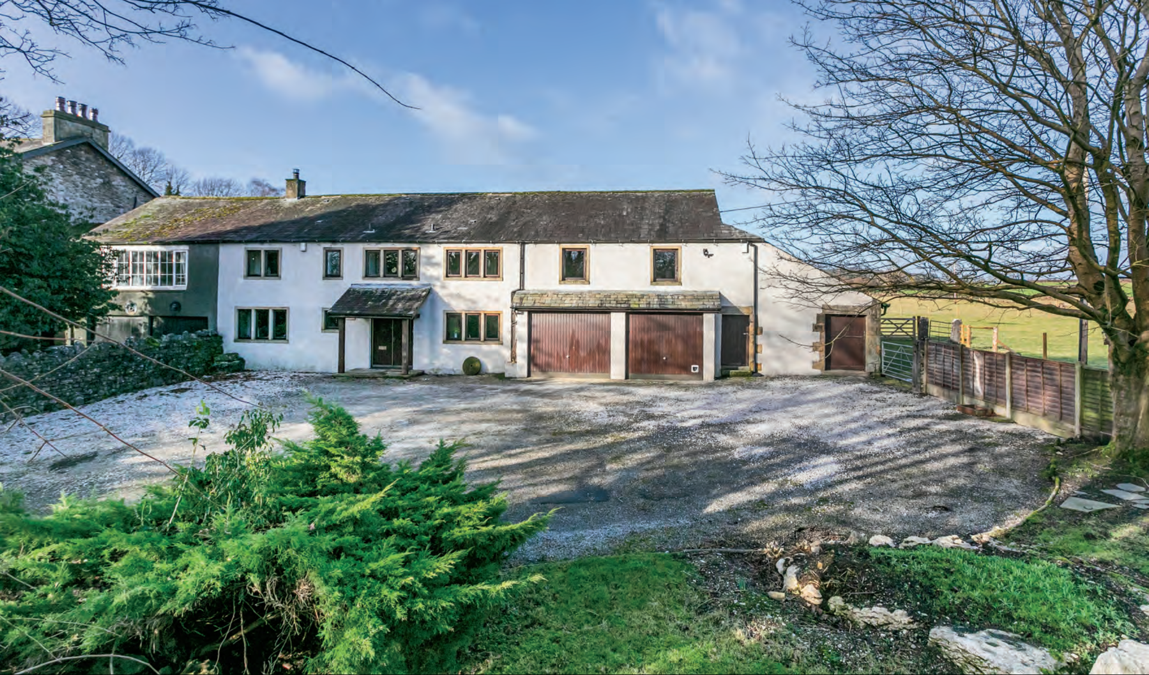
Dale House Barn Tewitfield | Lancashire | LA6 1JH
